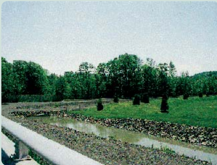
1. North Branford Stormwater Retention and Remediation Basin Project
