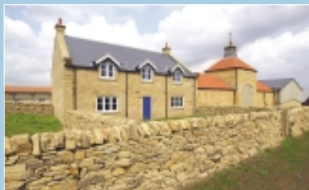
Waste water treatment works This attractive farm style building houses Scarborough's new, state of the art waste water treatment works. During construction over 30 quarries were investigated to obtain stone typical to that used in the surrounding area.
